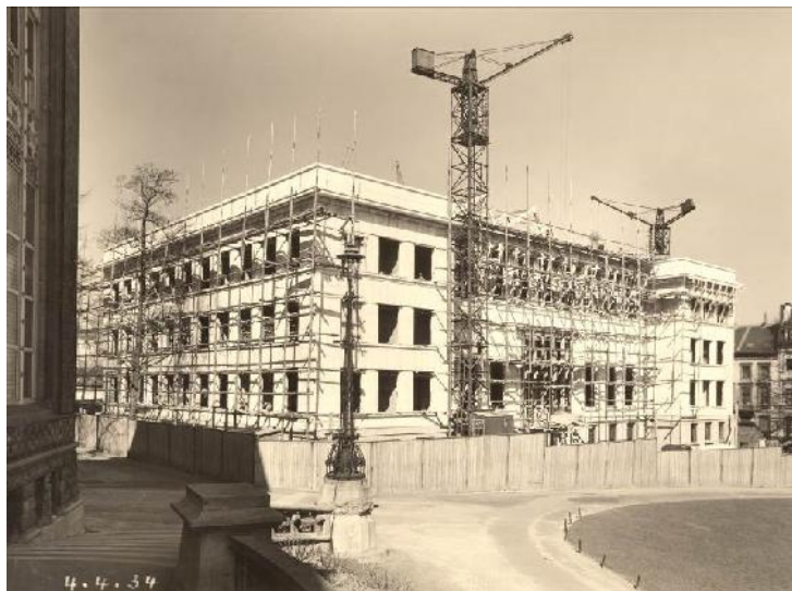
Figure 1 – Construction de l'Institut Eastman, 1934.
